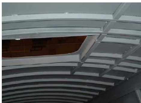
Before roof panelling
