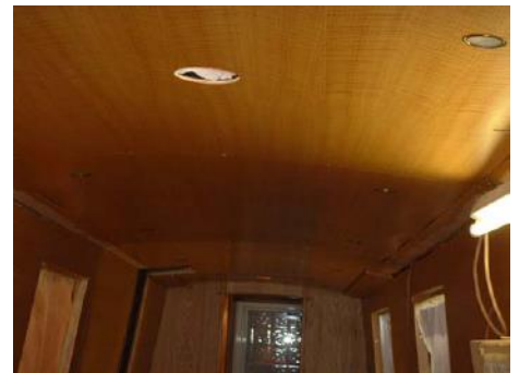
After roof panelling
