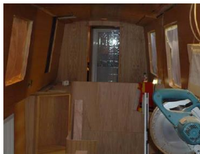
After the wall panelling
