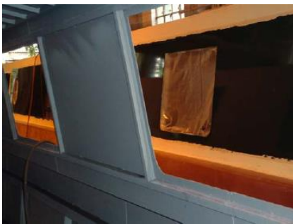
Before the wall panelling
