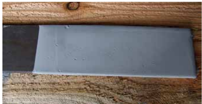
Excessive layer build up of ZINGA with pinholes
