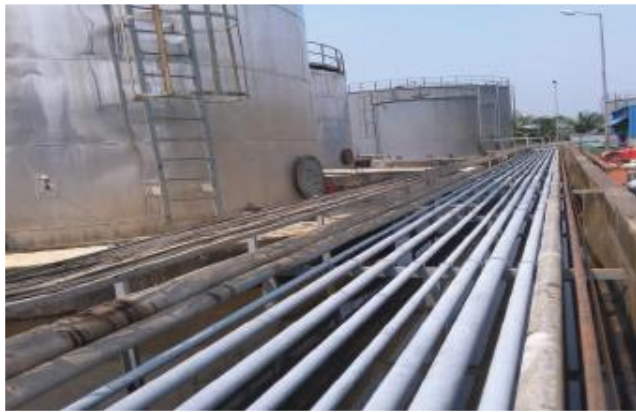
Application of PU topcoat 50 – 60 \mu\text{m} DFT & delivery to the client CLC POWER in November 2020
