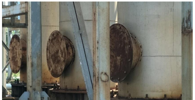
Condition before surface preparation & application of ZINGA
